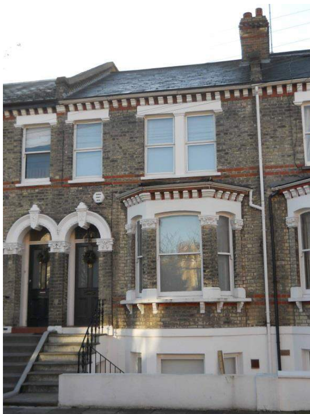
Nos. 25-45 Irving Road. Gault brick facades with red brick string courses. Note the distinct modillions under the eaves.
