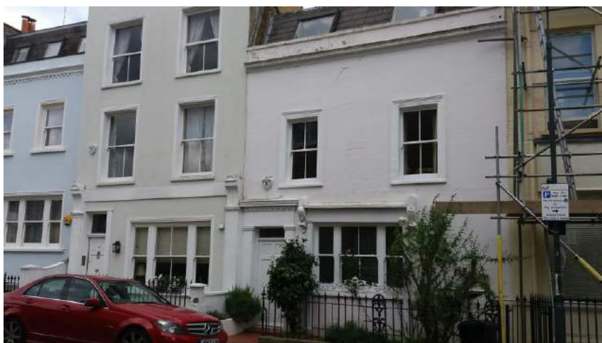
Nos. 71 and 73 Milson Road as they are now with retained pilasters and console brackets and cornices (no. 73 only).
