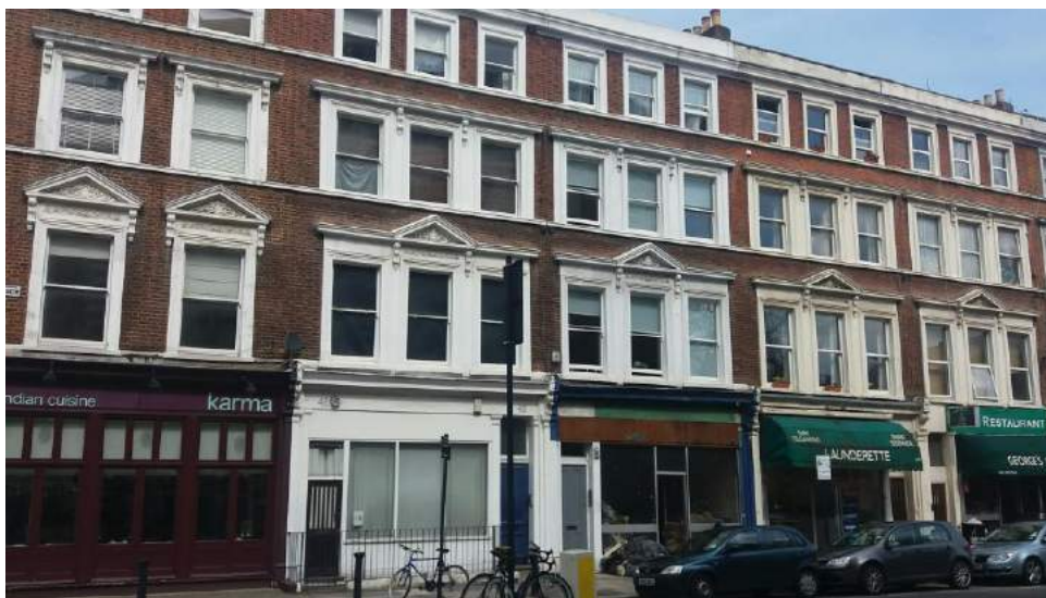
Pilasters, console brackets and cornices are largely intact. Nos. 2-12 Maclise Road.
