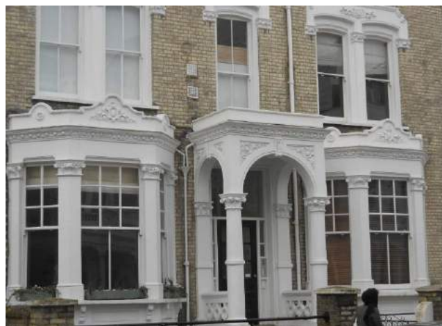
Elaborate stucco pediments on nos. 55 to 91 Sinclair Road.
