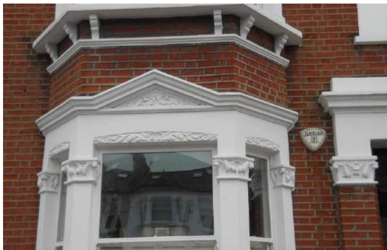
Stucco pediments and capitals on bays, Dewhurst Road east.
