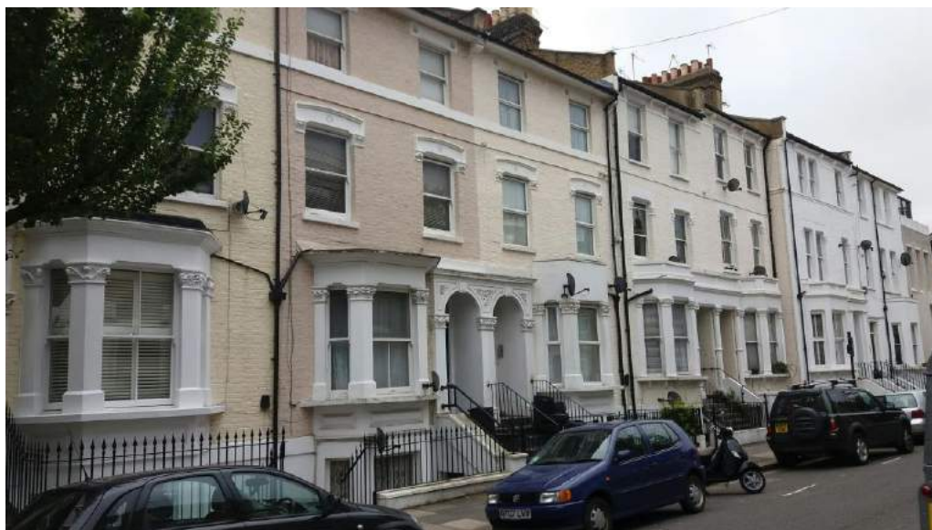
Nos. 107-121 Milson Road.
