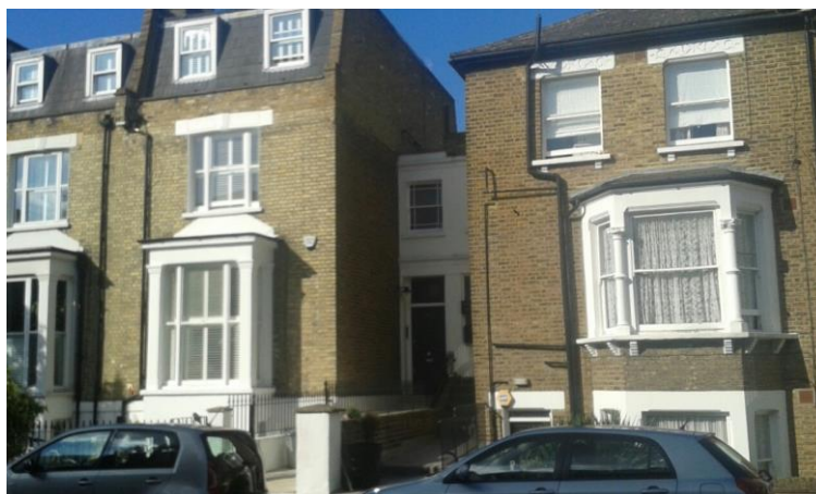
Paired villas with entrances in the recessed links.
