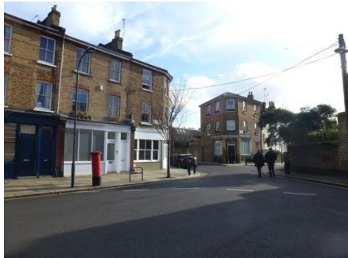
Former retail at ground floor of no. 20 Bradmore Park Road.
