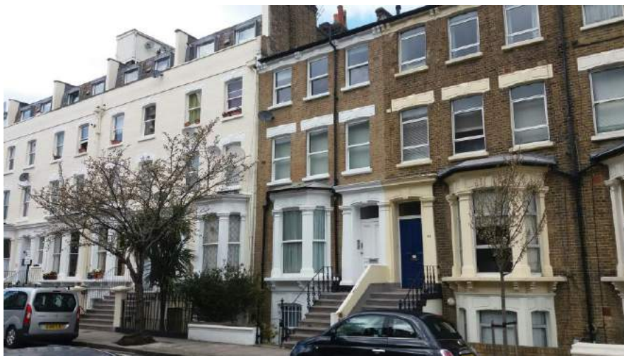
Nos. 48-56 Minford Gardens break the uniformity with mansard roofs and parapets.
