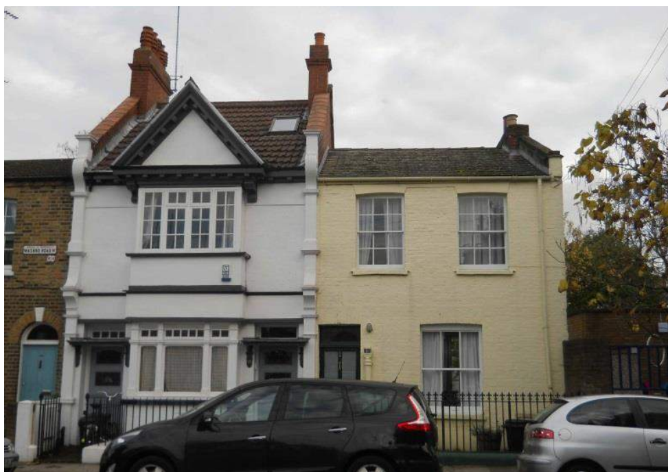
Unusual full height pilasters, no. 42 Masbro Road.
