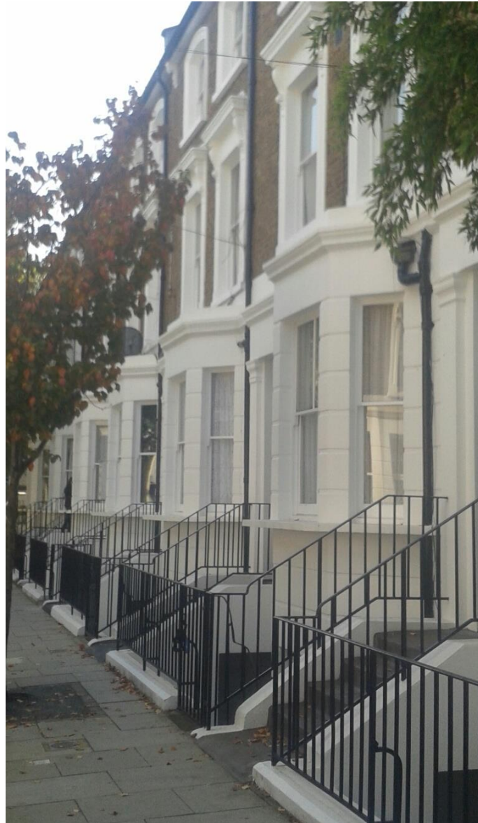
Nos. 1-13 have lost the original iron railings but fortunately the modern replacements are uniform in this group.
