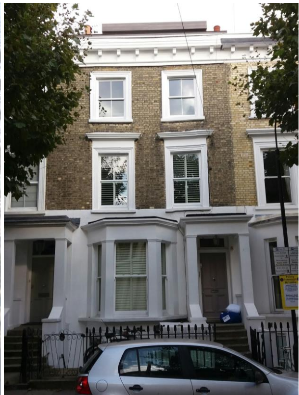
Restored cornice and modern roof extension behind the parapet, no. 21 Barclay Road.
