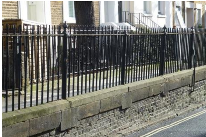
Original Victorian railings with stone plinths should be retained and restored as they give Cambridge Grove and Leamore Street its character and reinforce its sense of place.
