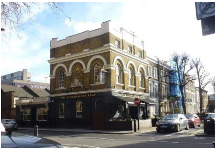
The Stonemasons Arms, formerly the Cambridge Public House, holds the corner of Cambridge Road and Glenthorne Road.
