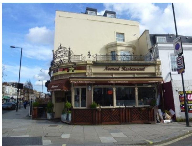
Now a restaurant, much of the character of the former Brackenbury Arms Public House remains.
