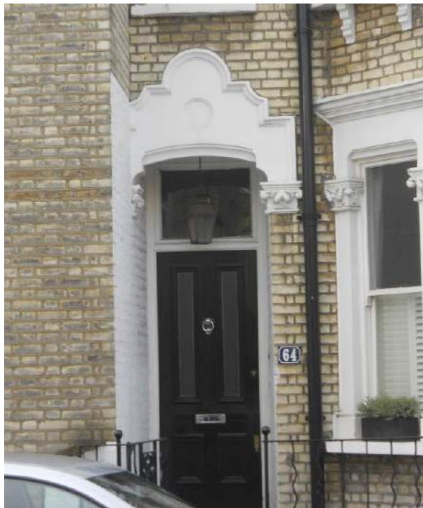
Elaborate stucco pediments, nos. 60-66 Milson Road.
