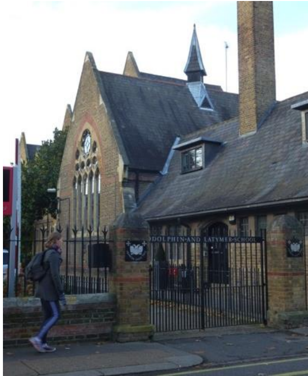
Godolphin and Latymer School – Iffley Road showing the original schoolroom (1862) with its ecclesiastical windows and fleche on the roof, behind the school keeper's lodge added in 1905. The dormer windows are modern.
