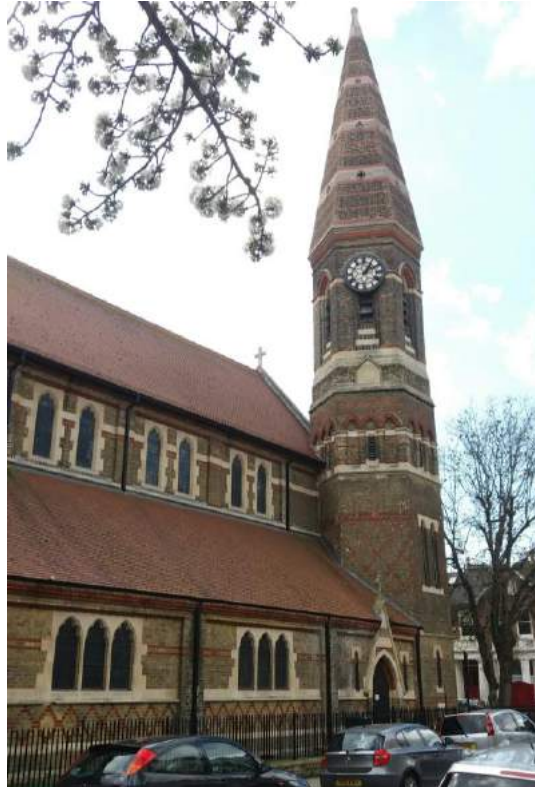
St. Simon's Church viewed from Minford Gardens.
