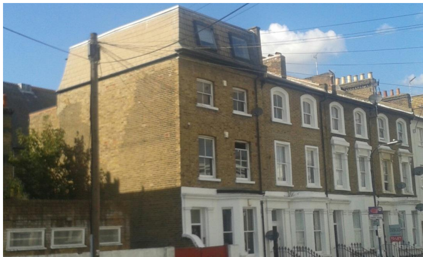
Missing architraves and an unsympathetic prominent mansard roof on no. 27.
