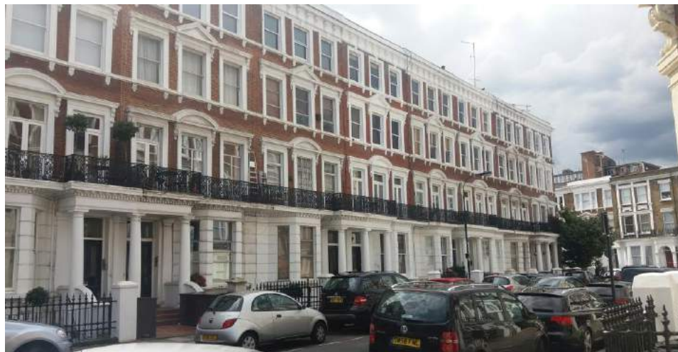
Nos. 33-47 Maclise Road.
