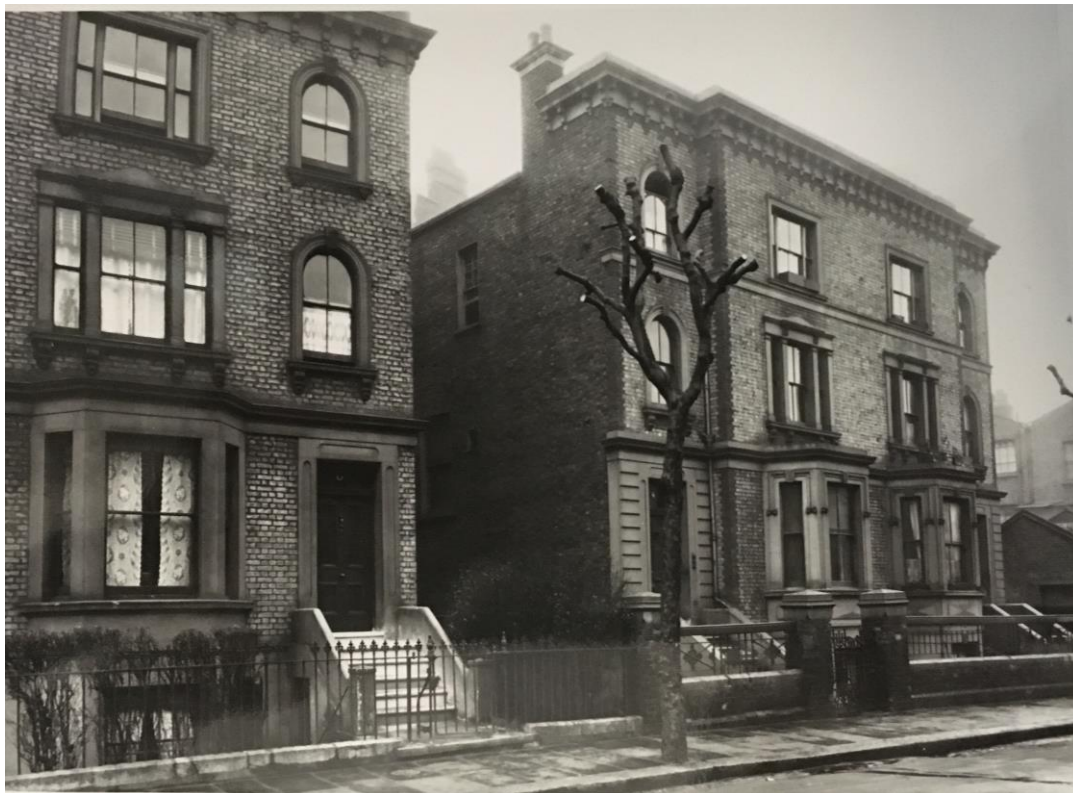
Nos. 2-6 photographed in 1931. The cornices are intact on nos. 2 and 4 and the original boundary wall and railings can be seen. (Photograph courtesy of LBHF Local Histories Library).
