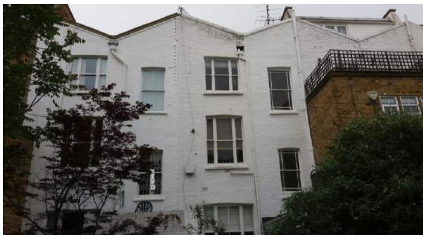
Prominent valley roofs, rear of Porten Road houses viewed from Ceylon Road.
