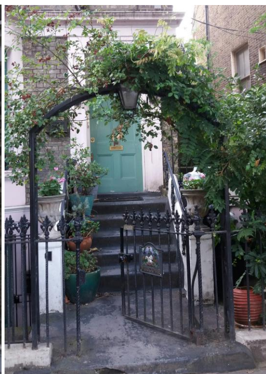
Non-original but sympathetic arched lamp holder, gates and iron railings, no.6 Barclay Road.
