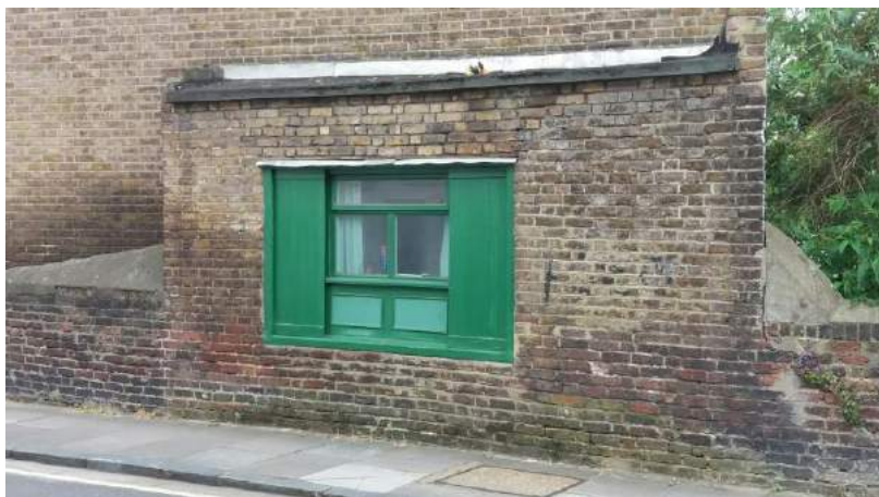
Serving hatch. Flank elevation of no. 1 Faroe Road on to Milson Road.
