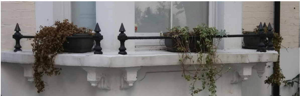
Original wrought iron window sill castings.
