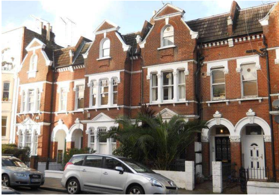
Houses in Addison Gardens, nos. 142-148. Richly detailed facades are further enhanced by planting in front gardens.
