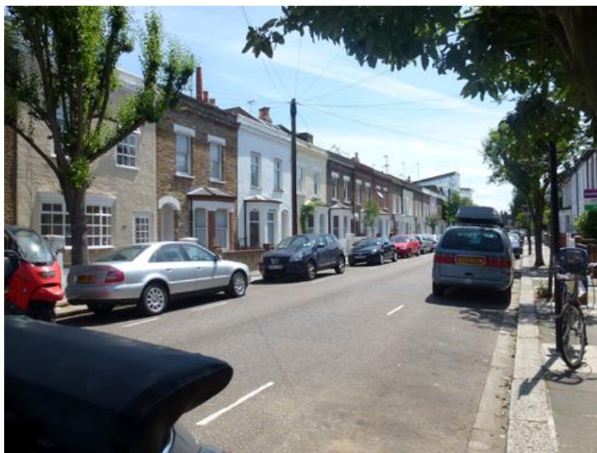
Nasmyth Street showing some unfortunate alterations; painted brickwork, a bow window on the ground floor of a flat fronted property.
