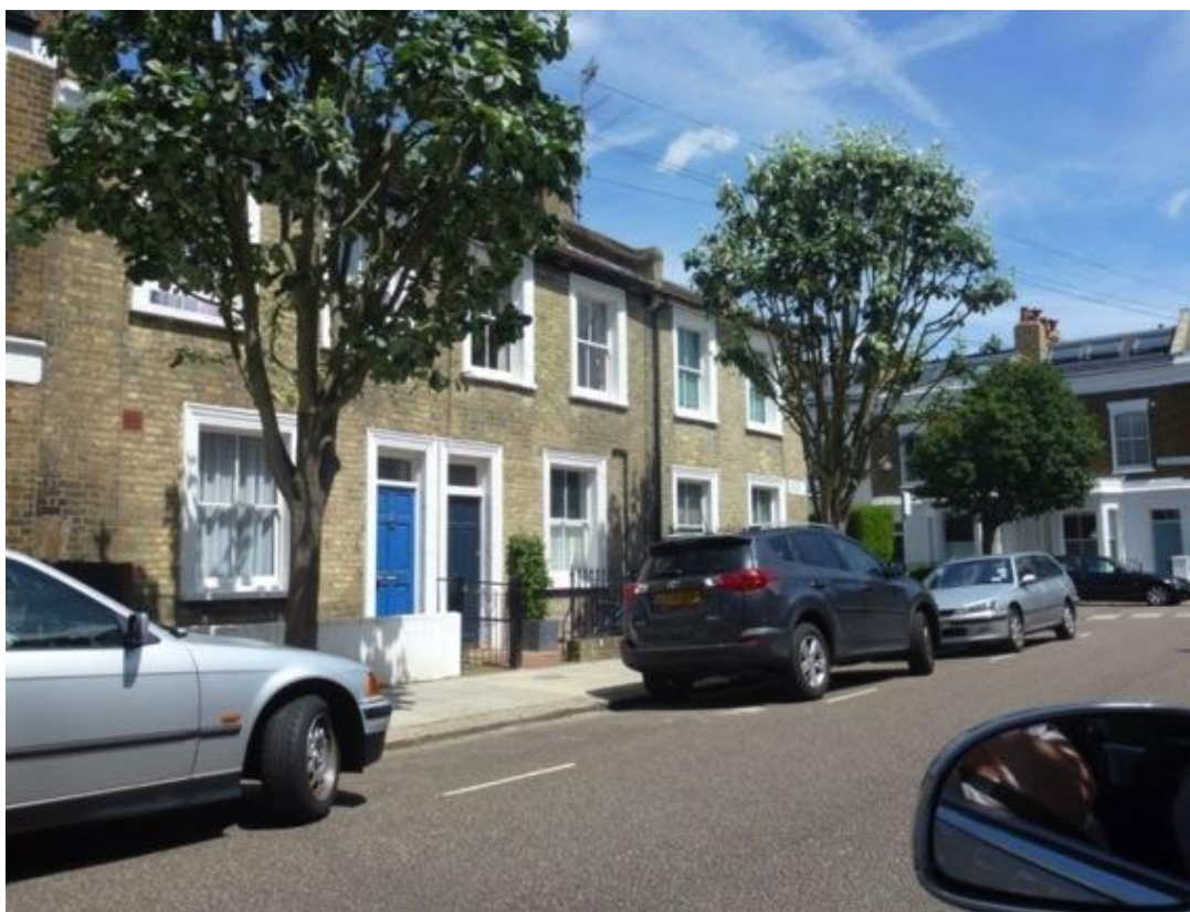
Two storey cottages in Furber Street – note the plaster mouldings around doorways and windows; timber sliding sashes and plain lights above solid six panelled timber doors. The neat simplicity and elegance of these mid-19 th Century cottages have been preserved and maintained.
