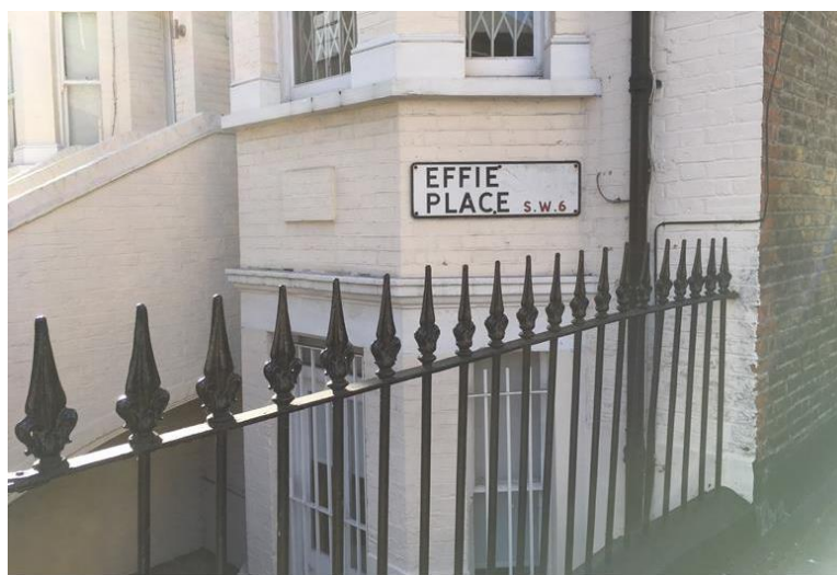
Bridge over lightwell to entrances and old street name plate. Effie Place.
