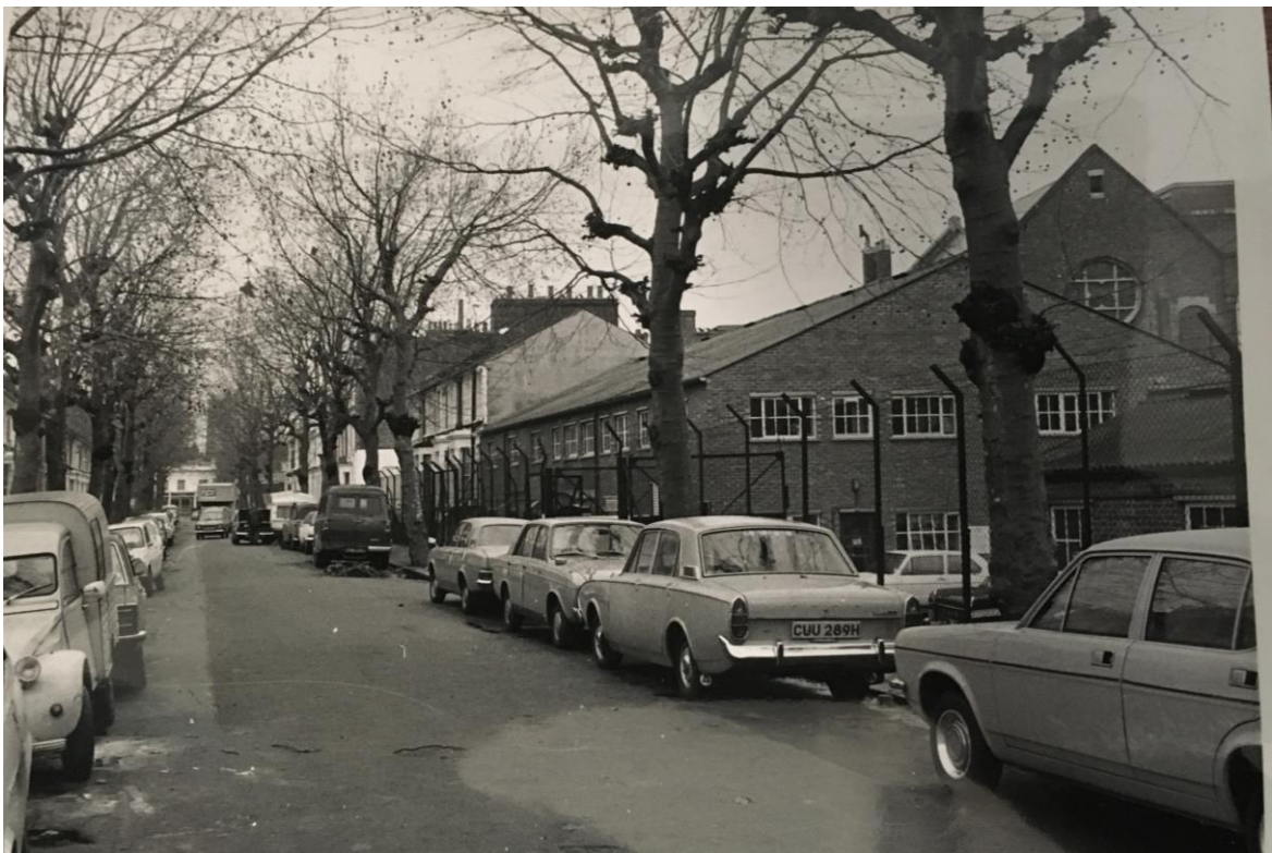
Council Depot, on site of demolished terrace nos. 37-57 Barclay Road, photographed in 1977, since demolished (photograph courtesy of LBHF Local Histories Library).
