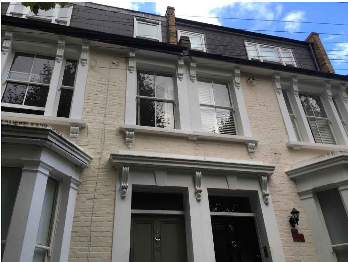
Distinctive console brackets under the eaves and cornices above entrances and around bays.
