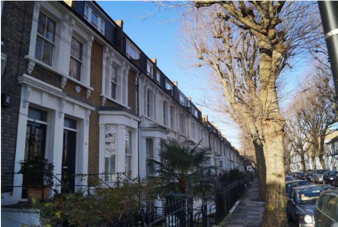
Nos. 50-56 (even) Barclay Road. Most premises have roof extensions.
