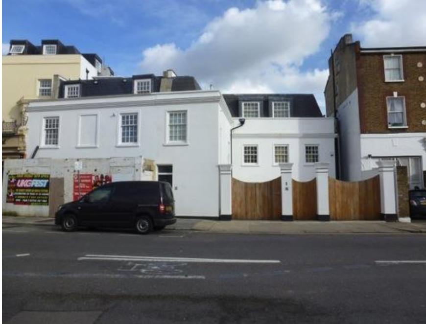
Nos. 1, 1a and 3 Brackenbury Road.
