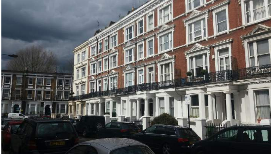
Nos. 14-26 Maclise Road.
