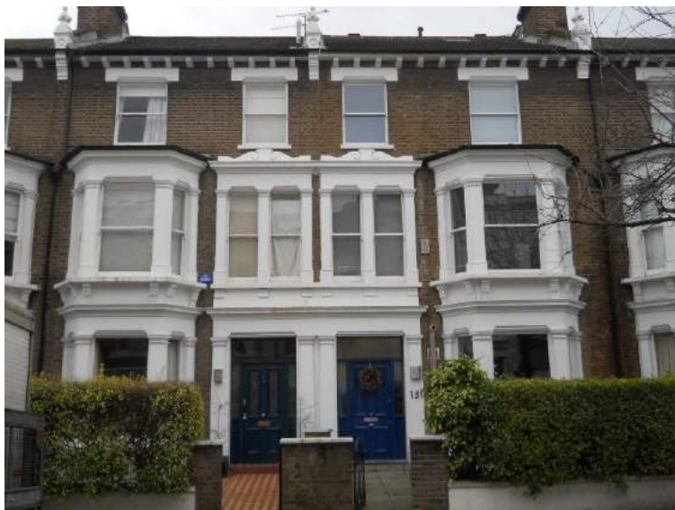
Paired windows above the entrances with stucco scrolled pediments. Nos. 145-161 Blythe Road.
