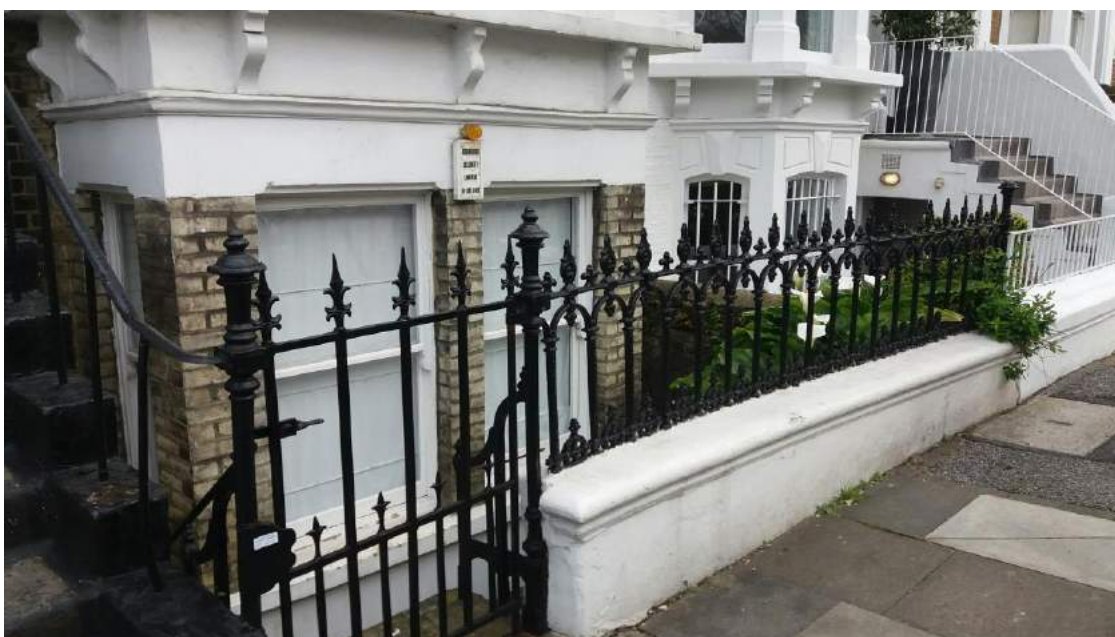
No. 73 Westwick Gardens, ornate iron railings intact.
