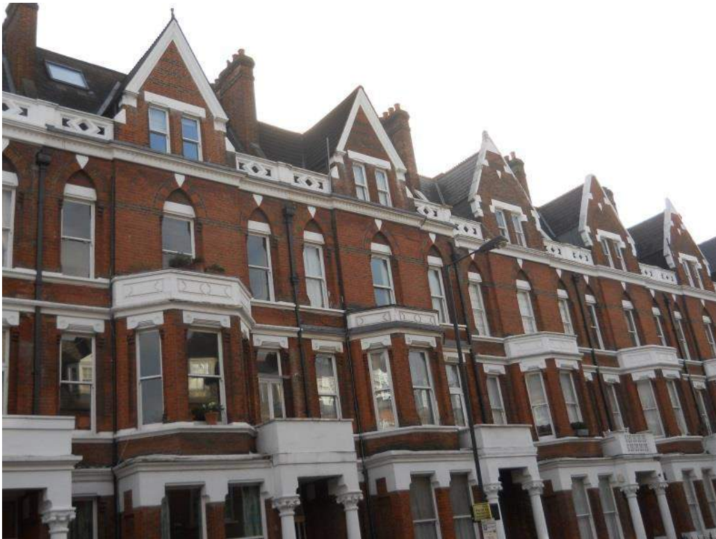
Nos. 29-51 Addison Gardens with prominent bays, gables, parapets and porticoes.
